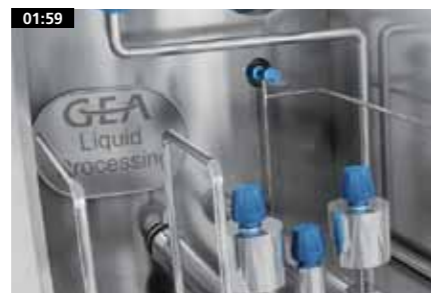
01:59 Silo tank agitator - CIP valve - GEA Liquid Processing design
